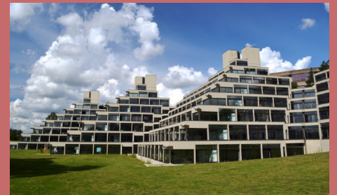
Credit Taken by John Fielding, Gery Balding and Kaysgeog
